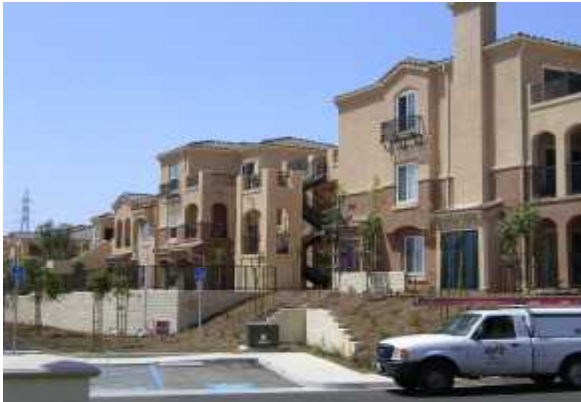
Figure 25: La Costa Paloma developed By Community HousingWorks and Mercy Housing California
