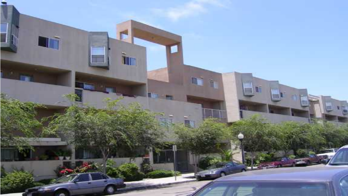
Figure 10: Hacienda Townhomes developed by San Diego Community Housing Corporation
